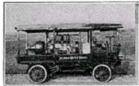
Thawing Outfit Mounted on Truck.
